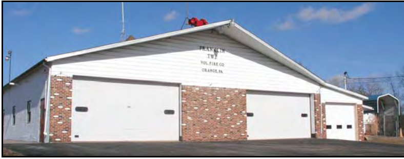
Franklin Township Fire Department
