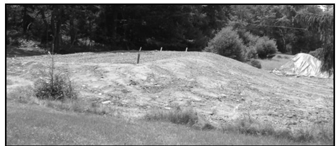
Sand Mound Under Construction
