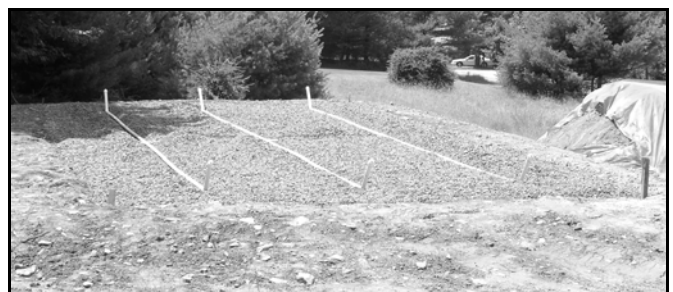
Sand Mound Under Construction
