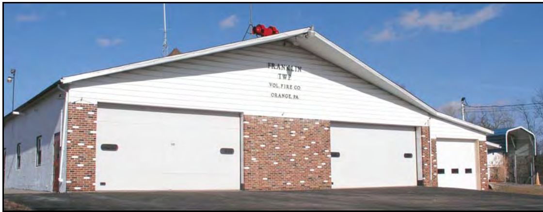
Franklin Township Fire Department
